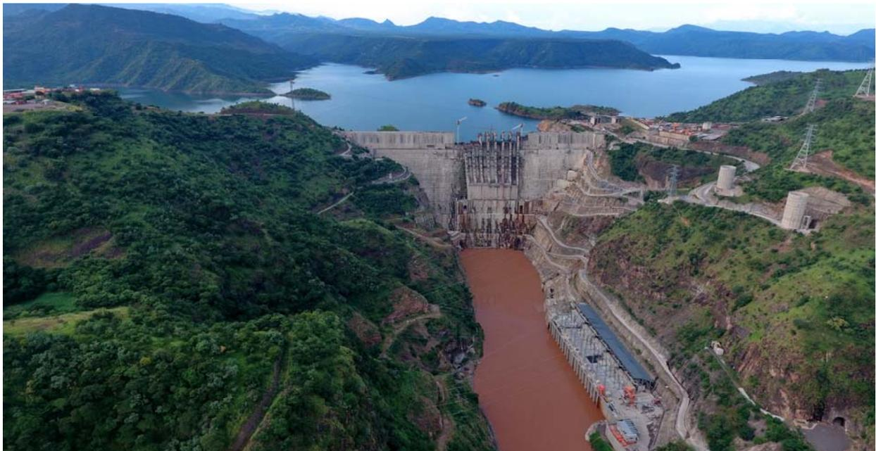
Fig. 1 View of the dam: the spillway is under construction and the reservoir reached 190 m over 250 m (July 2016)
