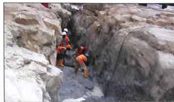
(b) Dental treatment along a large subvertical joint parallel to the riverbed.
