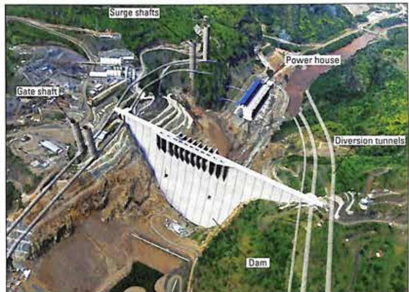
Fig. 2. The final layout adopted for Gibe III, showing: the dam crest spillway; and, the left bank powerhouse.
