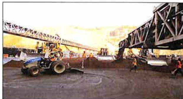
(g) Application of the bedding mix.
