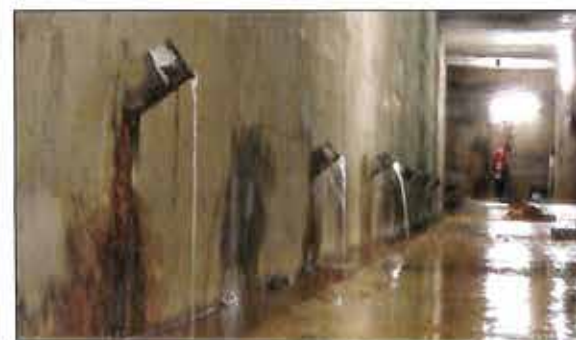
(c) Hot spring inflows conveyed inside the dam inspection gallery.
