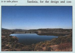
tural rehabilitation of the Eleonora d'Arborea alla Cantoniera di Busachi (Cantoniera) dam. The aim of the assignment is to improve the safety standards through the structural reinforcement of the lateral segments, ensuring full use of the reservoir's water resources, the company announced in early November. Cantoniera is a 100 m-high buttress concrete gravity dam located on the Tirso river, near Busachi
