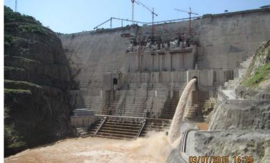
Fig. 6 Wet Commissioning of Left Middle Level Outlet ( $Q \approx 300 \text{ m}^3/\text{s}$ )
