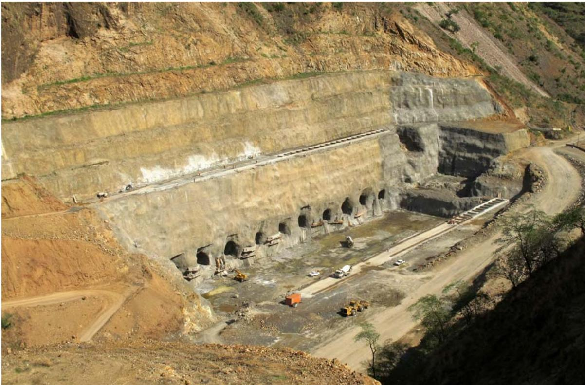
*Fig. 2. Panoramic view of the Power House excavation front during concreting*
