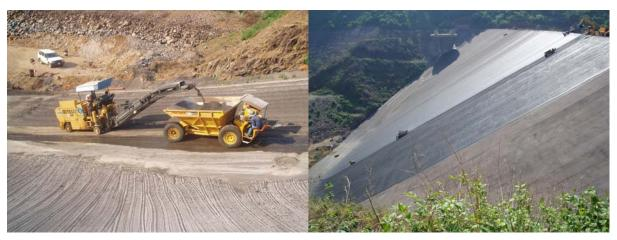
Figure 6–Rehabilitation works of the asphalt concrete facing
