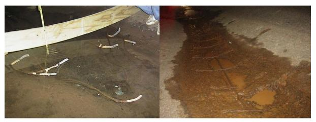
Figure 4-Erosion along tunnels invert zones
