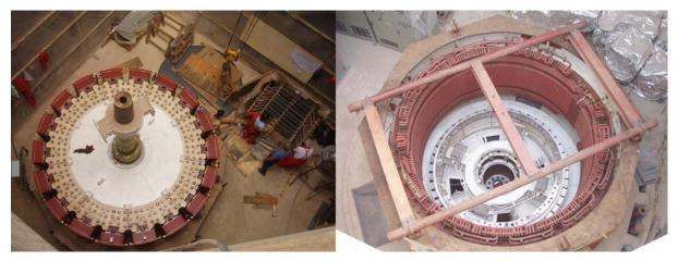
Figure 8-Assembly of generator rotor and stator after rehabilitation
