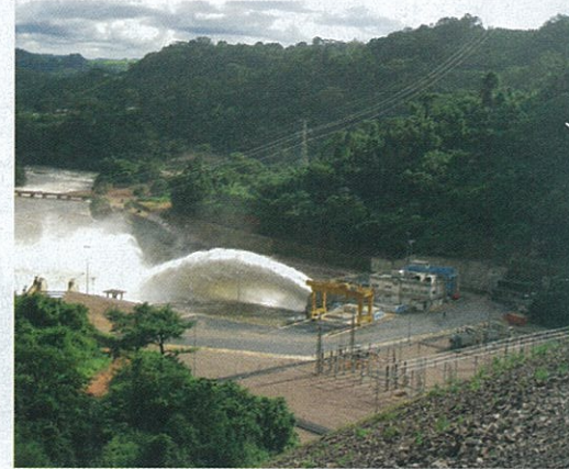
Above: Figure 5 – Semi-outdoor powerhouse located at the dam toe (Bumbuna, IP=50MW).
