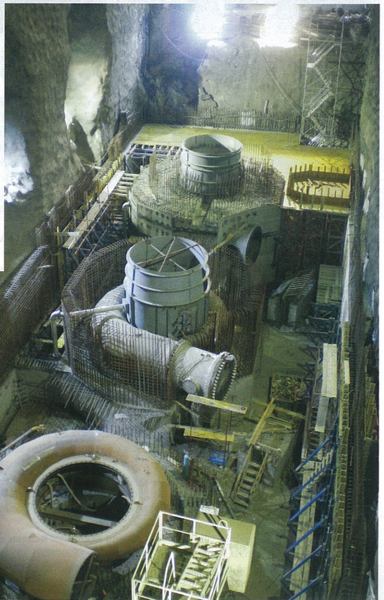
Below: Figure 7 – Underground powerhouse during construction (Beles, IP=460 MW)
