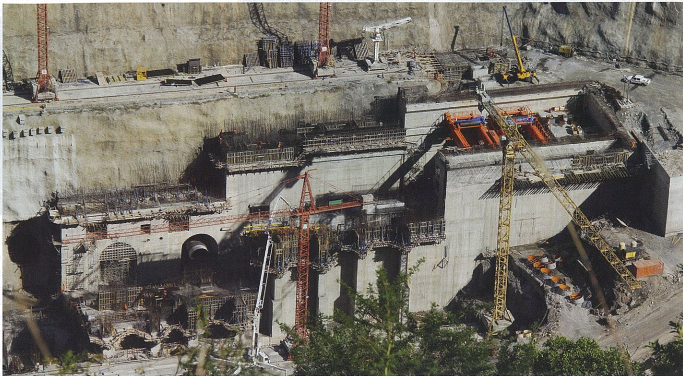
Above: Figure 8 – Large semi-outdoor powerhouse under construction (Gibe III, 1870MW.) Left: Figure 9 – Design of the huge Grand Ethiopian Renaissance HPP ( IP=6000MW).
