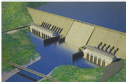
Above: Figure 8 – Large semi-outdoor powerhouse under construction (Gibe III, 1870MW.) Left: Figure 9 – Design of the huge Grand Ethiopian Renaissance HPP ( IP=6000MW).
