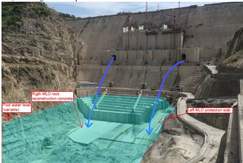
Fig. 4: MLO pool upstream protection, before impounding.
