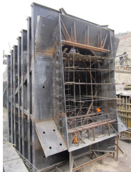
Fig. 5: Inlet block stiffening structure
