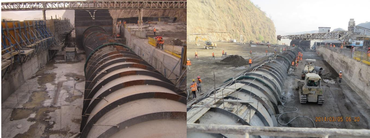
Fig. 11: RCC recess and subsequent pouring around Right Middle Level Outlet, March 2014
