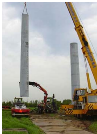
Figure 11 – Erection of shaft
