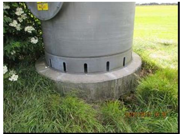
Figure 4 – 400kV line pylon foundation, Denmark
