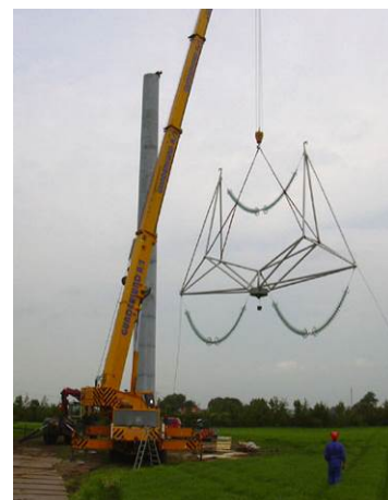
Figure 13 – Lifting lattice top
