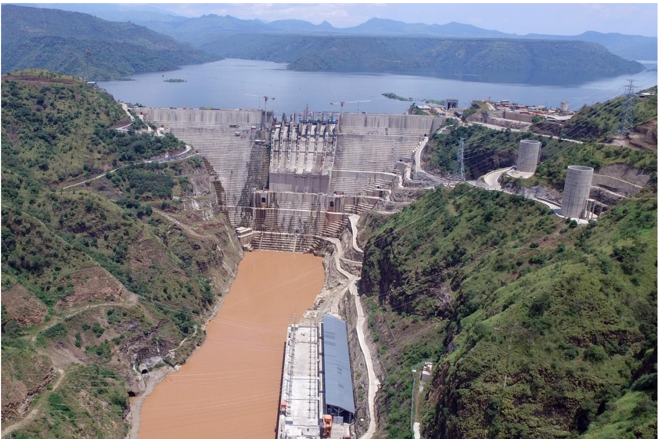
Fig. 1: Gibe III plant in operation, while spillway construction is under completion, October 2016
