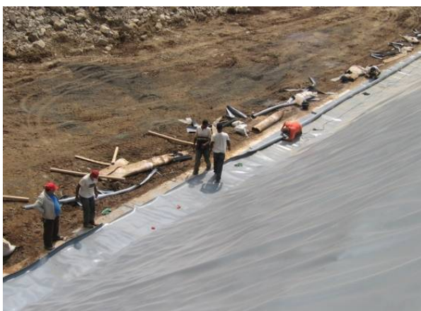
Figures 8 and 9. At left, the PVC geomembrane installed over a completed dam section is watertight welded onto the PVC geomembrane protruding 2 m from the crest of the section below. At right, placement of the fill for the fourth Section of the cofferdam
