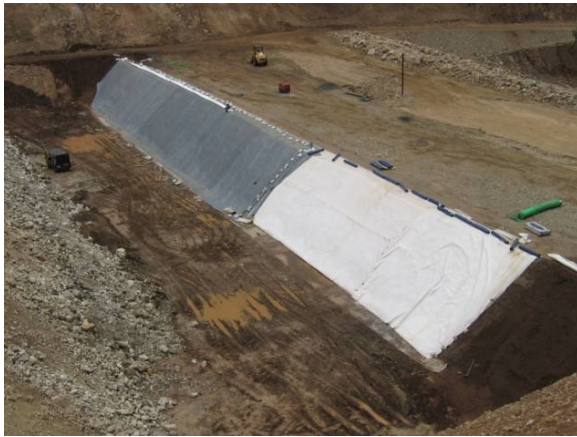
Figures 6 and 7. At left the first section of the cofferdam is completed, the first anti-puncture geotextile (white) is placed on the sand layer, and the PVC geomembrane (gray) is placed over it. At right, construction of the second section starts after the second anti-puncture geotextile has been placed over the PVC geomembrane
