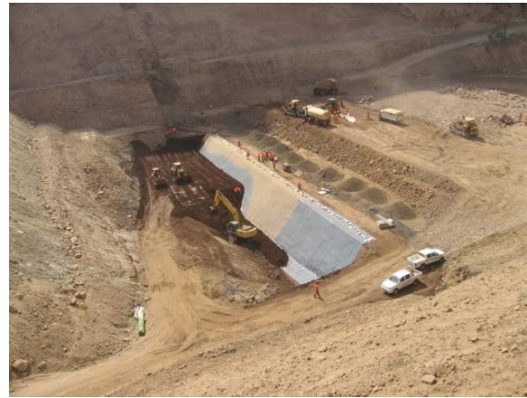
Figures 6 and 7. At left the first section of the cofferdam is completed, the first anti-puncture geotextile (white) is placed on the sand layer, and the PVC geomembrane (gray) is placed over it. At right, construction of the second section starts after the second anti-puncture geotextile has been placed over the PVC geomembrane
