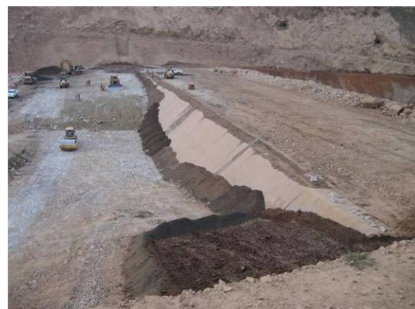
Figures 8 and 9. At left, the PVC geomembrane installed over a completed dam section is watertight welded onto the PVC geomembrane protruding 2 m from the crest of the section below. At right, placement of the fill for the fourth Section of the cofferdam
