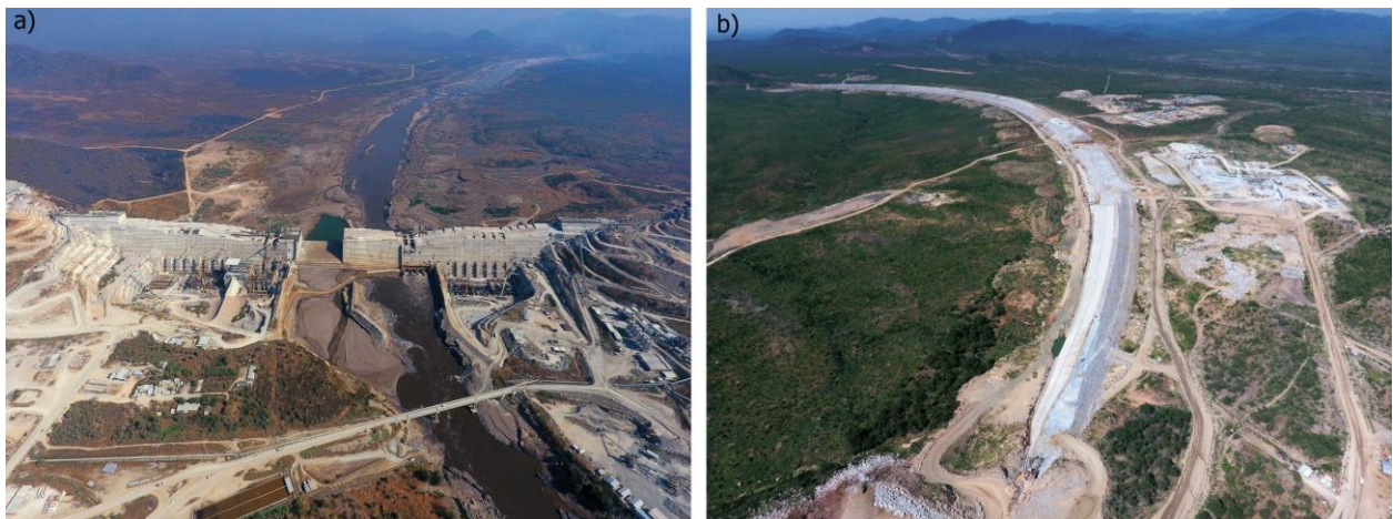
Fig. 2. a) RCC Main dam and b) CFRD Saddle dam views.
