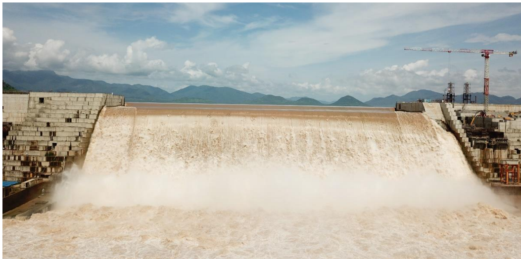
Figure 2 – GERdp hydroelectric project, Main Dam temporary stepped spillway.
